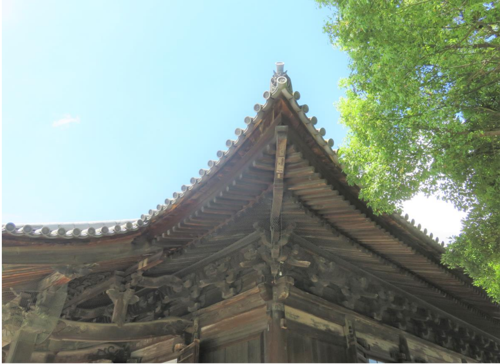
軒は二軒の繁垂木
