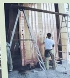
大扉の銅板設置工事 Copper plate construction of the large door
