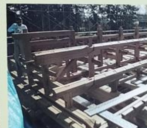
渡櫓の屋根工事 Construction of the Yagura ceiling
