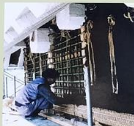
土塀の左官工事 Plastering of the earthen walls
